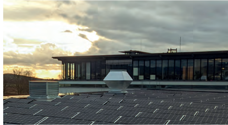
PV array on the roof of the new center for electrical energy storage in the Haid industrial area of Freiburg.
