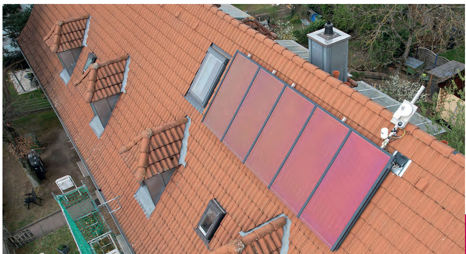
Pilot installation with colored solar thermal collectors in Freiburg St. Georgen.
