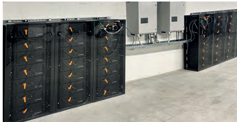
Multi-functional battery storage: Intermediate storage of PV electricity to optimize self-consumption and to flatten load peaks.
